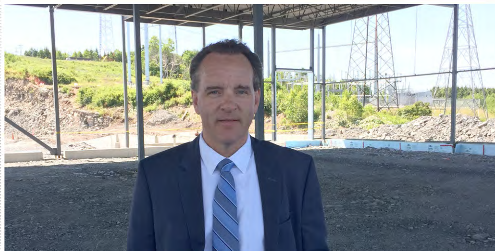
Construction is underway at East Point, where a new Sobeys location is scheduled to open in mid-2016. A spokesperson for the company said the grocery store chain would be pulling out of McAllister Place. PHOTO: KELSEY PYE/TELEGRAPH-JOURNAL
