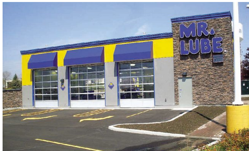
Mr. Lube is one of four new businesses to join the East Point Shopping family in 2014. PHOTO IS COURTESY OF MR. LUBE
