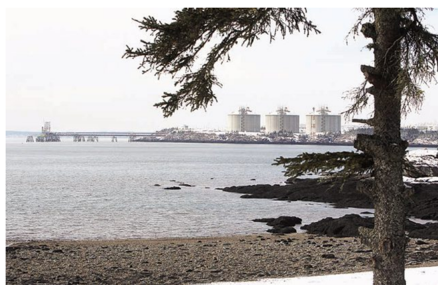
The Canaport LNG terminal is seen from Mispec Beach.
